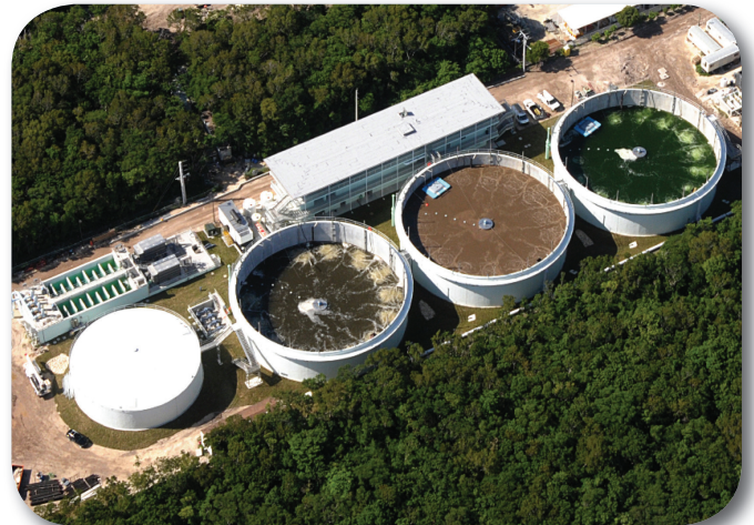
Aerial of Key Largo WWTD after its upgrade with the AquaSBR ® system, AquaDisk ® filters and IntelliPro ® system.
